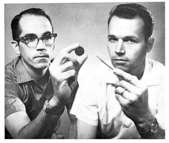
NEW SAPPHIRE GAGE, which can measure shock wave pressures approximately five times more powerful than those measured by similar gages, is displayed by its developers, R. A. Graham, left, and G. W. Ingram (both 5133).
